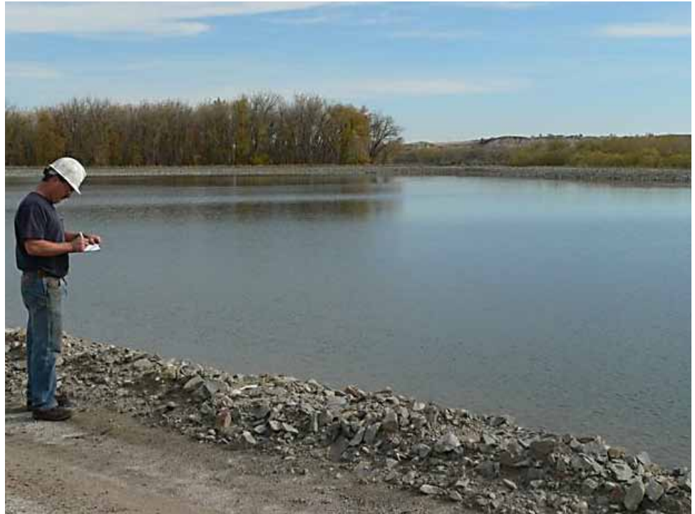
(Picture 6 – Lewis & Clark Station employee conducting an inspection of the Bottom Ash Pond.)
