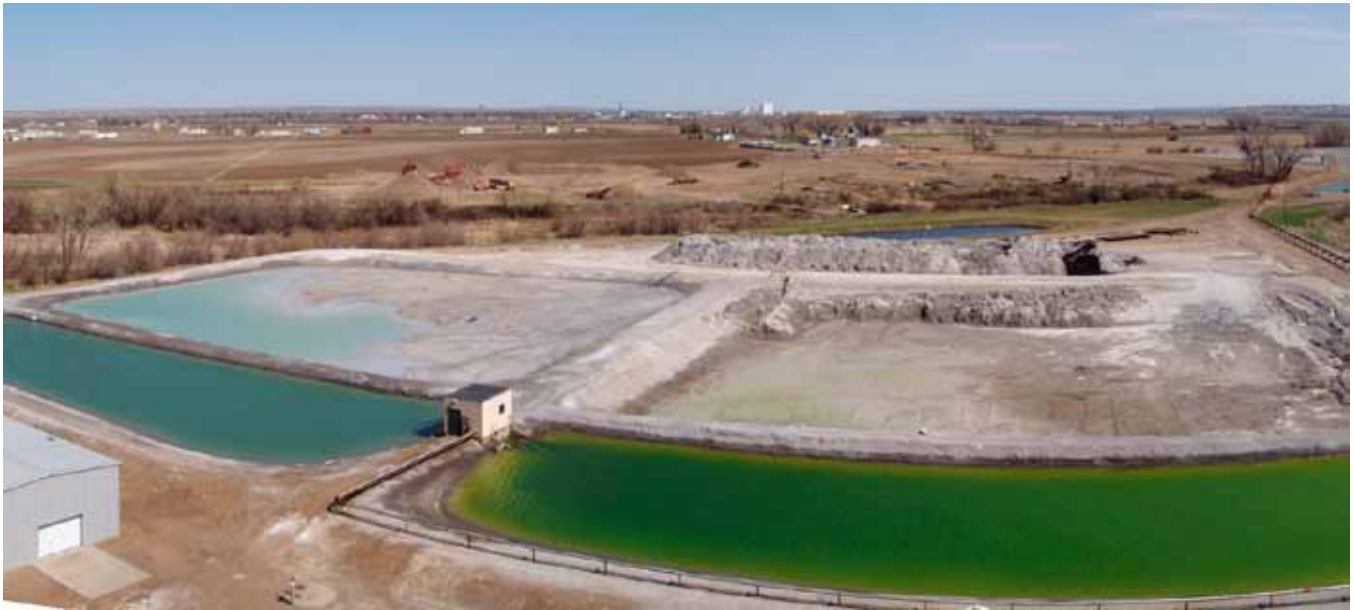
(Picture 11 – Lewis & Clark Station Scrubber Ponds showing the process of cleaning out the right pond in order to transition ash sluicing from the left pond to the right pond. Ash stockpiled on the HDPE-lined dewatering pad in the background.)
