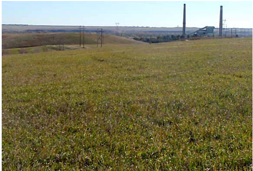
(Picture 9 – R.M. Heskett Station Active Ash Landfill Cap on Slots 1 through 5.)
