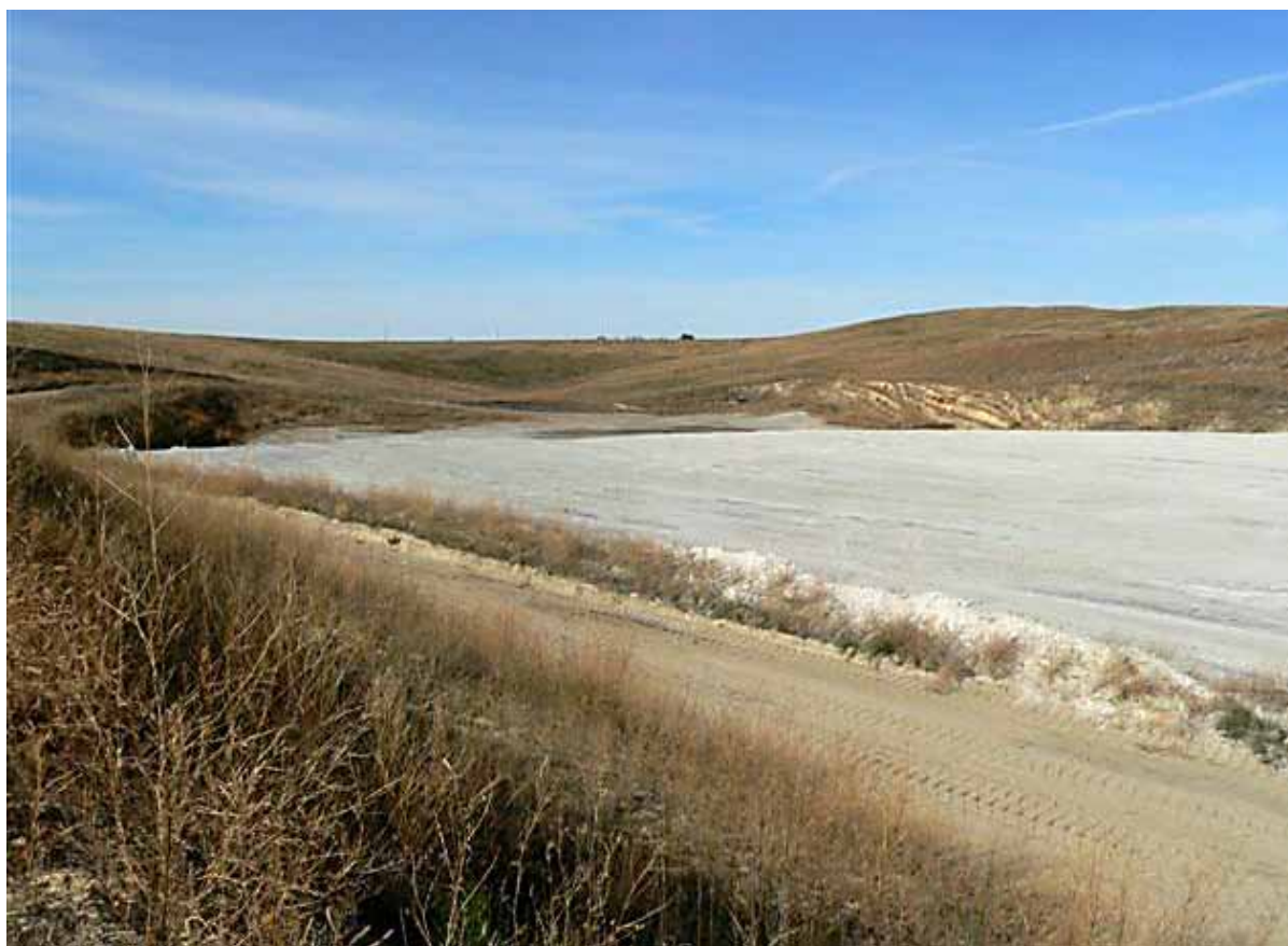
(Picture 8 – Savage Ash Landfill, where dewatered fly ash and bottom ash that are not beneficially used and FGD ash from Lewis & Clark Station are placed for permanent disposal.)
