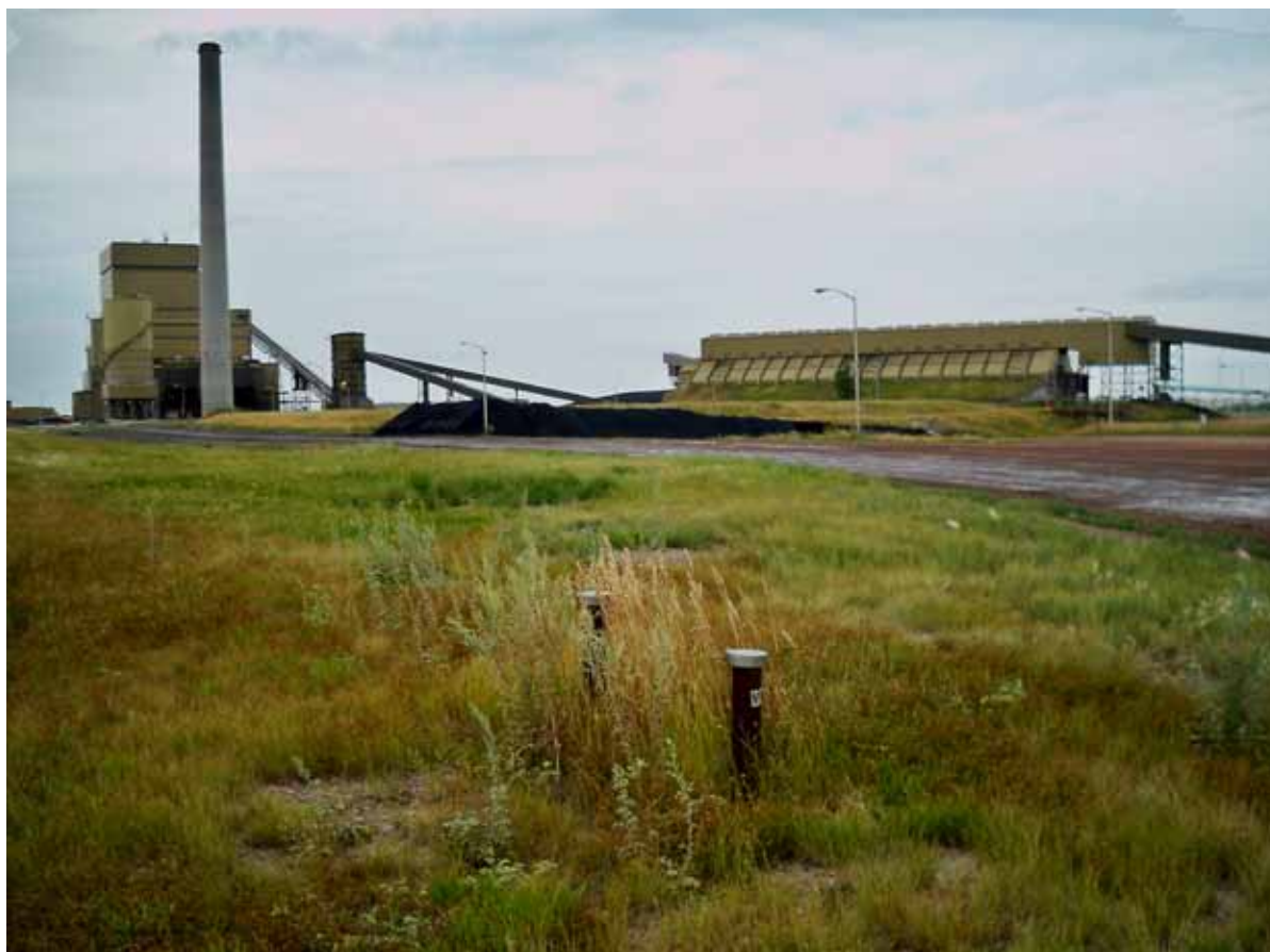
(Picture 10 – Groundwater monitoring wells in foreground at Coyote Station.)
