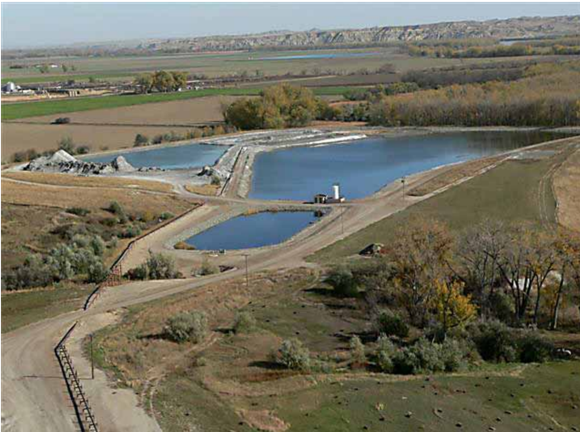
(Picture 5 – Lewis & Clark Station's Bottom Ash Pond (two cells in background) and smaller Wastewater Treatment Pond in foreground.)
